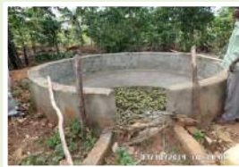
Fig. 10: Water harvesting structure for supplementary irrigation during dry spell
